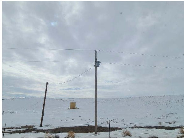
Photo 18 View of on-site AST and former oil and gas operation.
