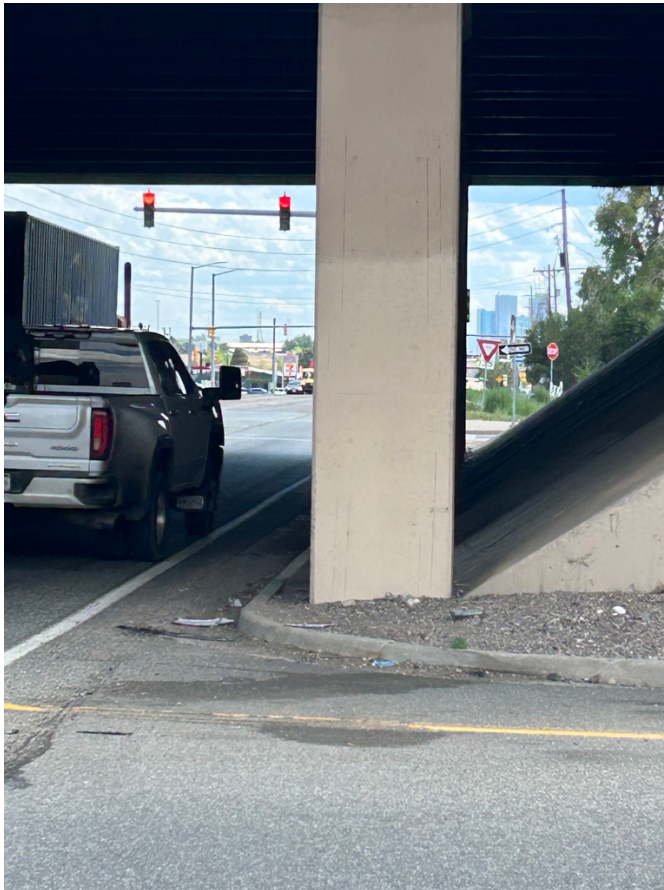
Figure 9 West side of Broadway Highway 36 underpass. This intersection is also the on ramp from I-25 south bound to Highway 36. July 30, 2026
