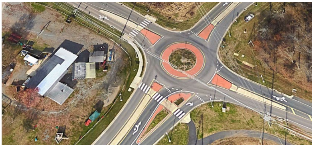
Roundabout, Fairfax County, VA
