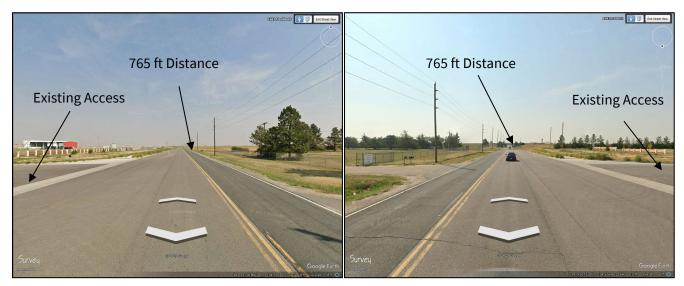
Figure 3. Entering sight distance. Left picture from the existing access facing north. Right from the existing access facing south.
