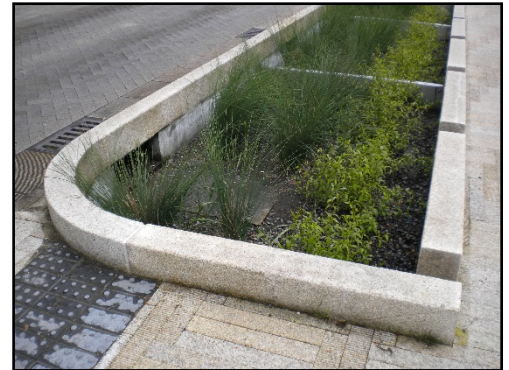
Fig. 3-27-BB: LID stormwater management feature
